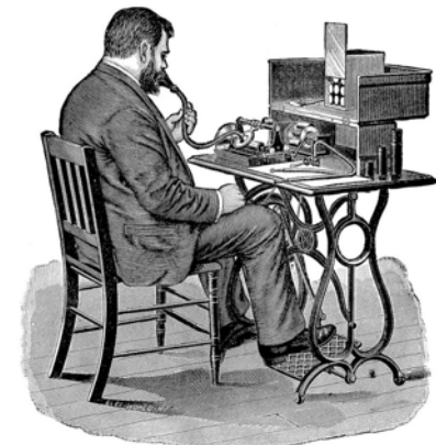
Fig. 4.—Graphophone, 1887, as Used in Receiving a Dictation and for Transcribing.
